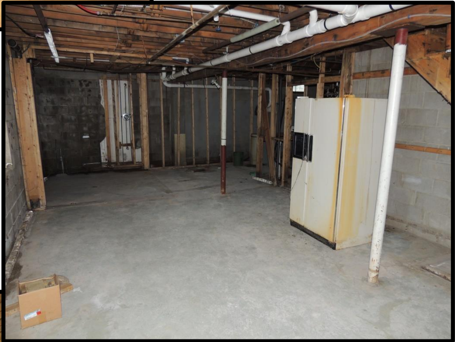
Large Unfinished Basement
